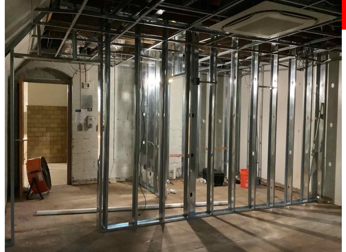
Interior wall framing at area B
