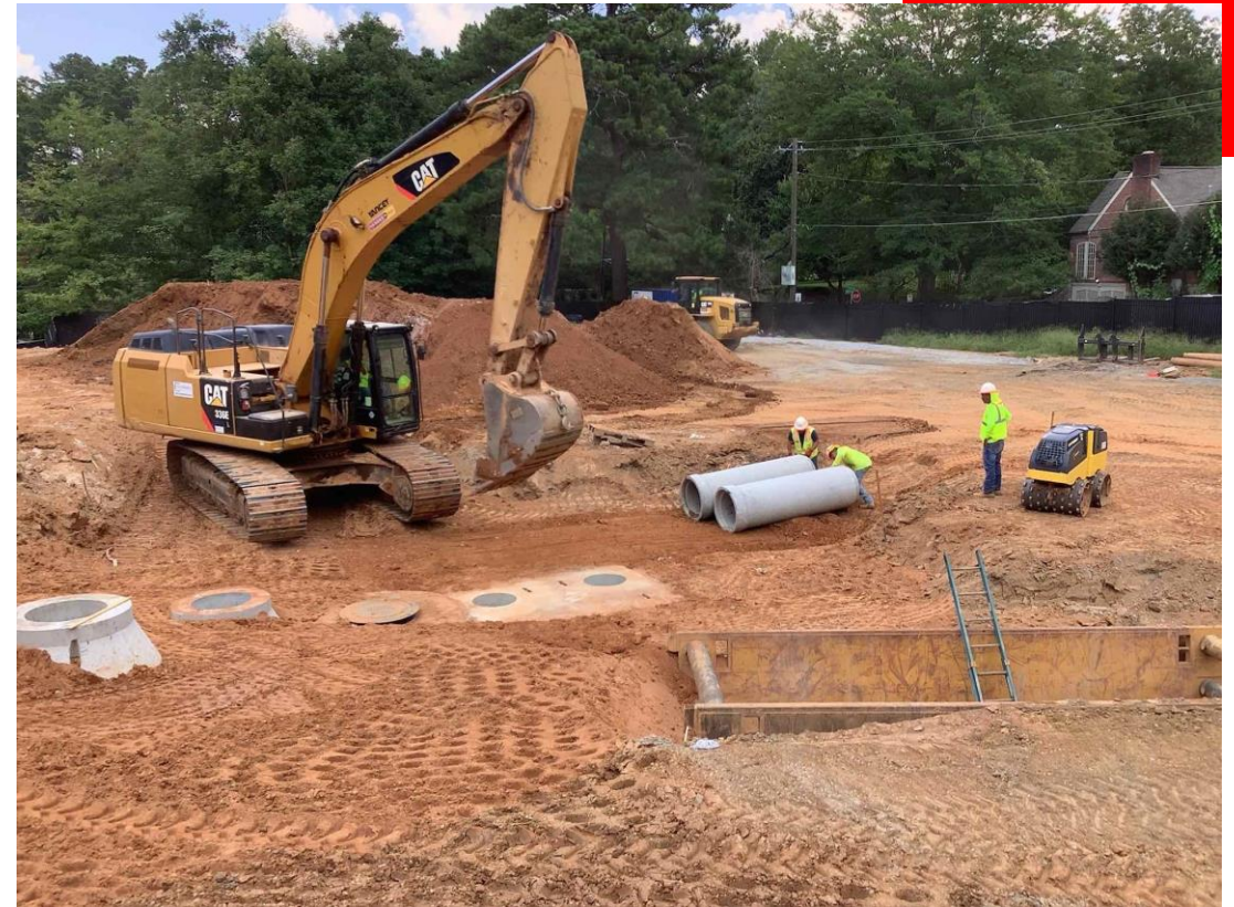
Site storm structure installation
