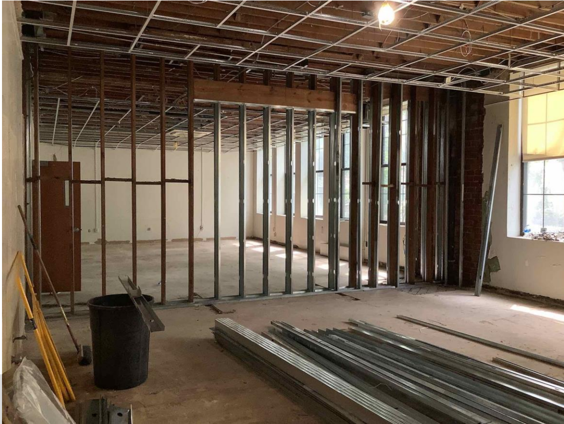
Interior wall framing at area B
